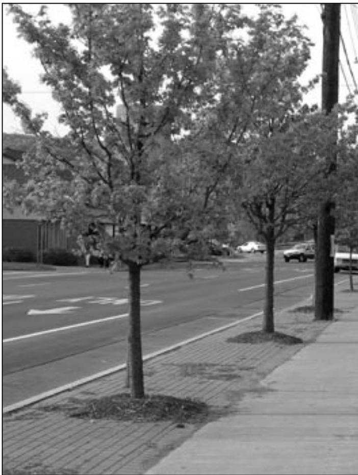
These *Acer campestre* have grown for nine years in a trench of CU-Structural Soil overlaid with un-mortared concrete pavers. Although when these trees were planted, we only used 15" of CU-Structural Soil in a continuous trench under the brick pavers, we now believe that 24" should be the minimum depth of structural soil, appropriate for smaller trees, while 36" is preferable in order to maximize rooting space and water availability.
